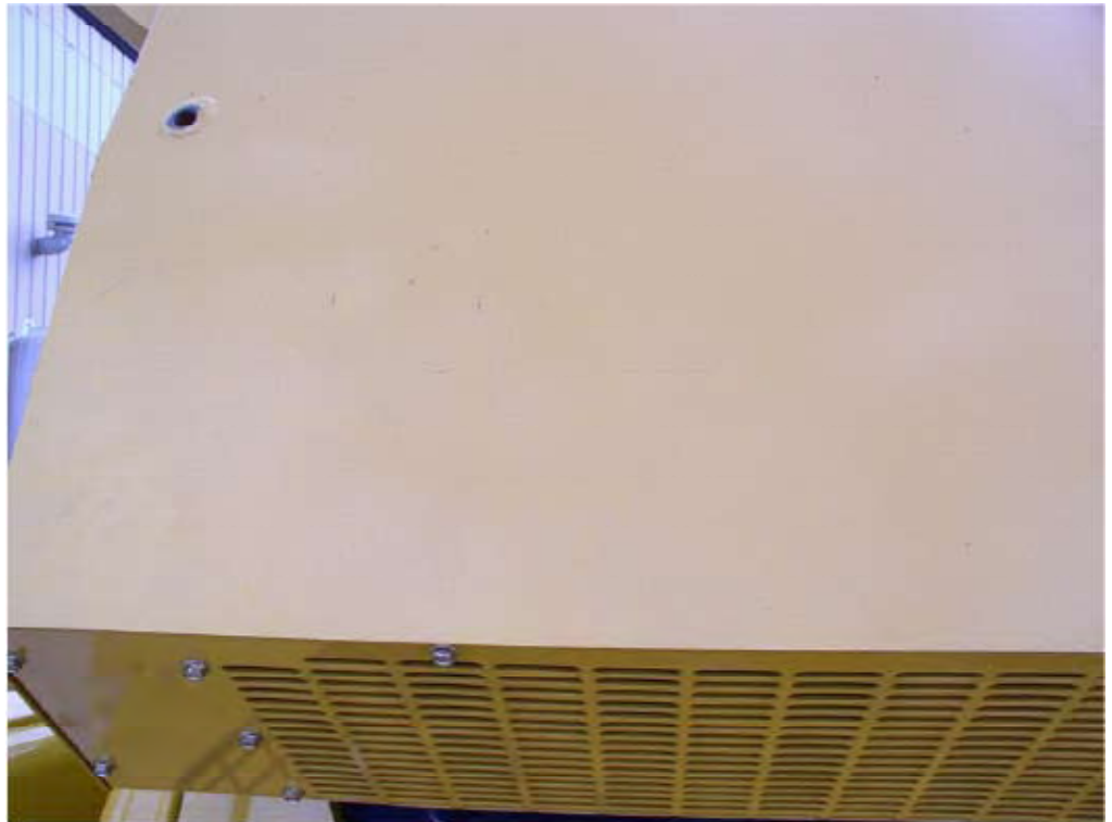
Figure 1: Cab top and rear view of roof.
