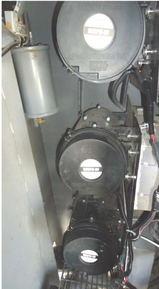
Fresh Air Intake Three RESPA-CF Units
