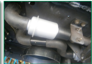
Rerouted Scavenger Lines
