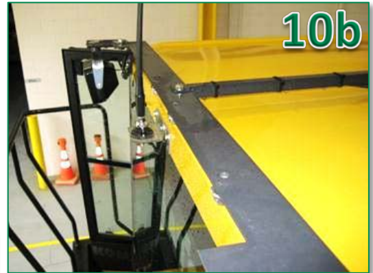
Beacon light bracing can be used to route wiring towards rear of cab.
