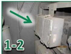
2. Remove the fresh air filter clamping systems from fresh air boxes (3).
